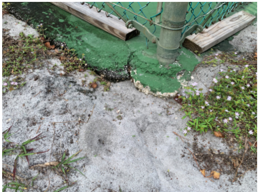
These photos show some of the erosion happening due to weakened sod not being able to recover from tire damage.
